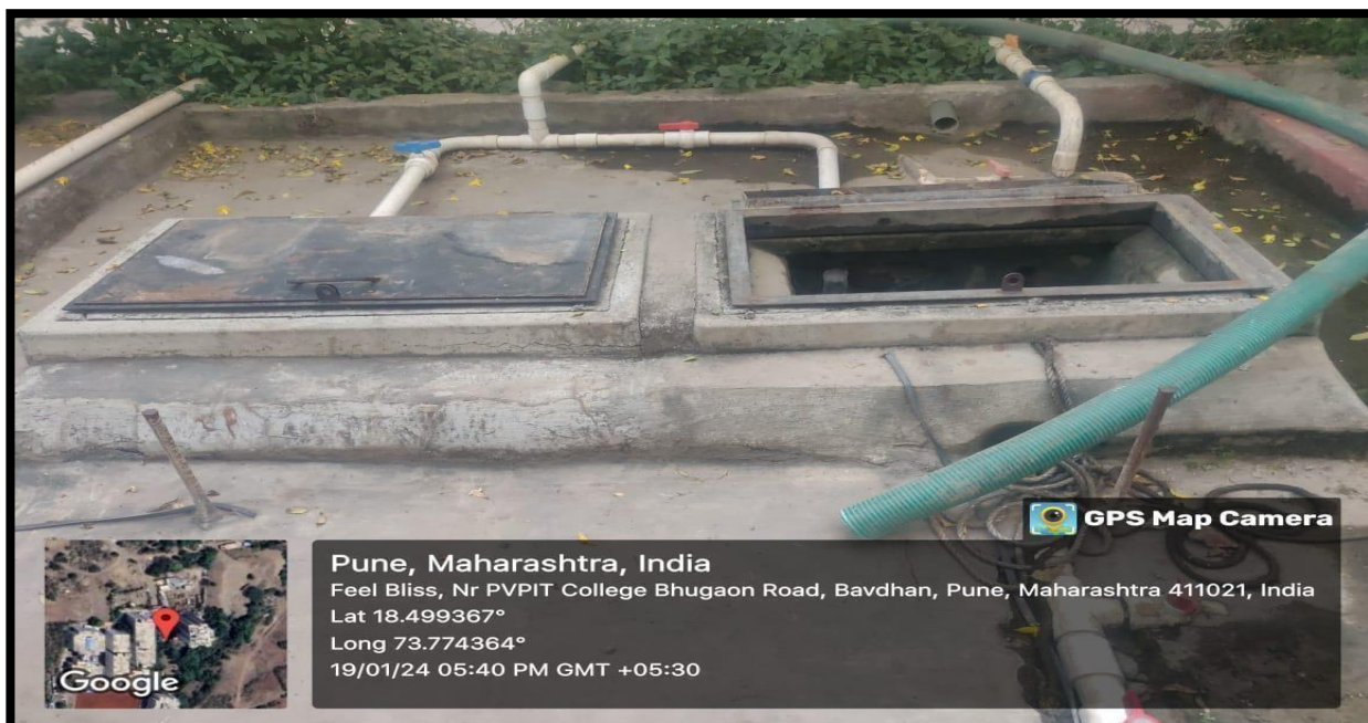
Construction of water storage tank near main gate of PVPIT College
